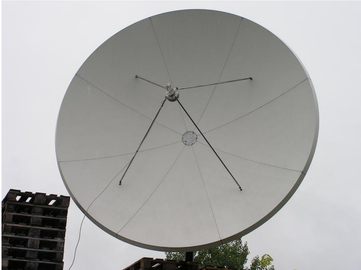
PF Prodelin 3.7m at ChinaStar 1 at 87,5°E_ C SPOT _
