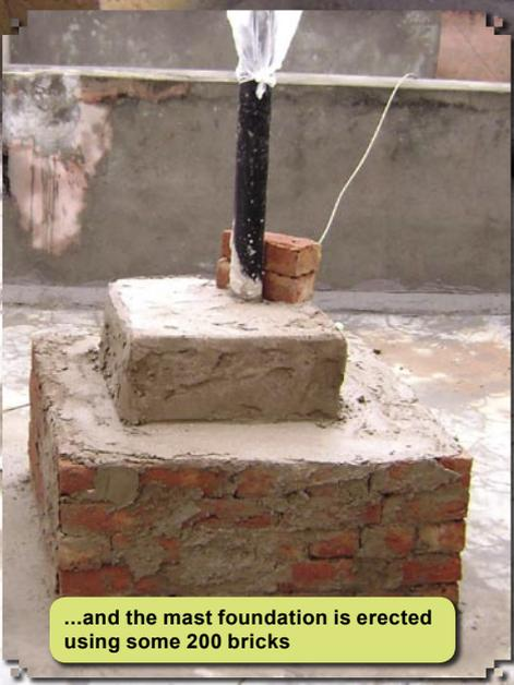
...and the mast foundation is erected using some 200 bricks
