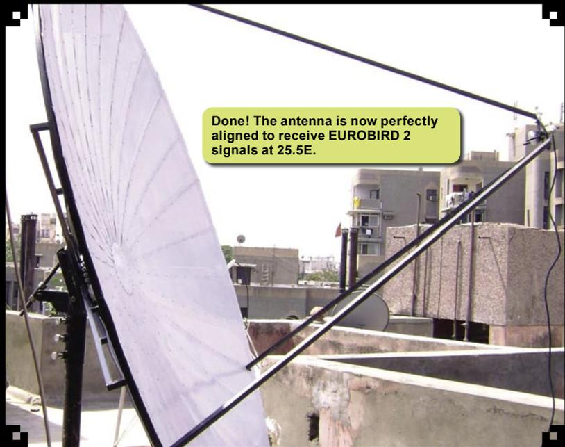
Done! The antenna is now perfectly aligned to receive EUROIRD 2 signals at 25.5E.
